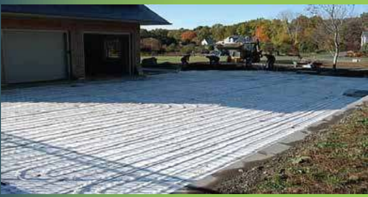
Snow Melt System Before
